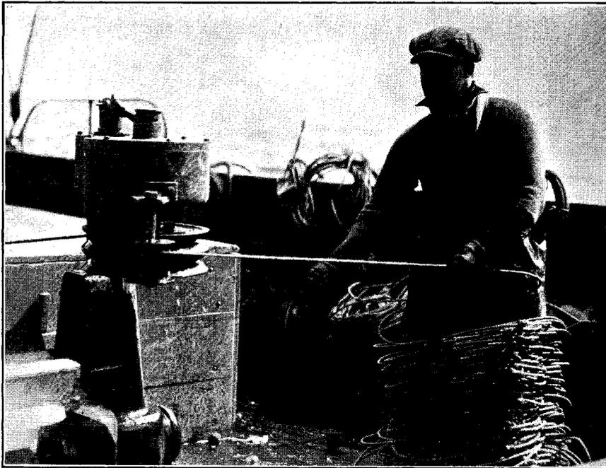
FIGURE 23.—The powered gurdy which pulls the line in over the roller, while the fisherman coils. Photograph by Ernest Pegler.
